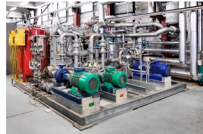
HIPA cooling circuit with recovery
